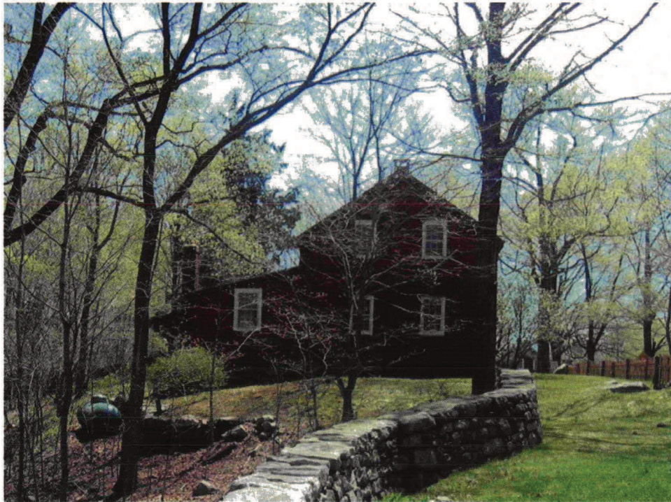
View south of the caretaker's house, 2003 (OCLP).
