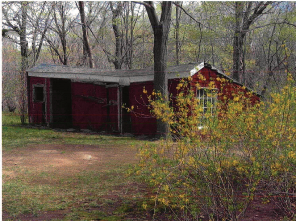
View northeast of the caretaker's garage, 2003 (OCLP).
