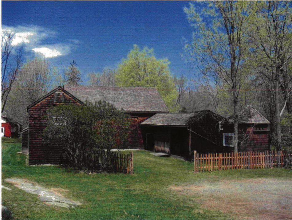
View north of the Weir/Young barn, 2003 (OCLP).
