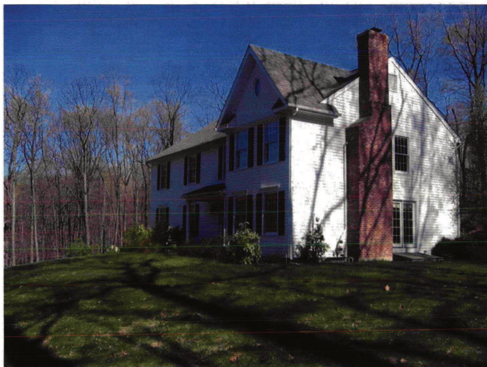
View southeast of the Westervelt house, 2003 (OCLP).
