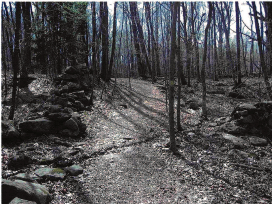
View west of stone lined ditch diverting water from a small stream (right side of path) across the footpath leading to Weir Pond and into an adjacent wetland, 2003 (OCLP).
