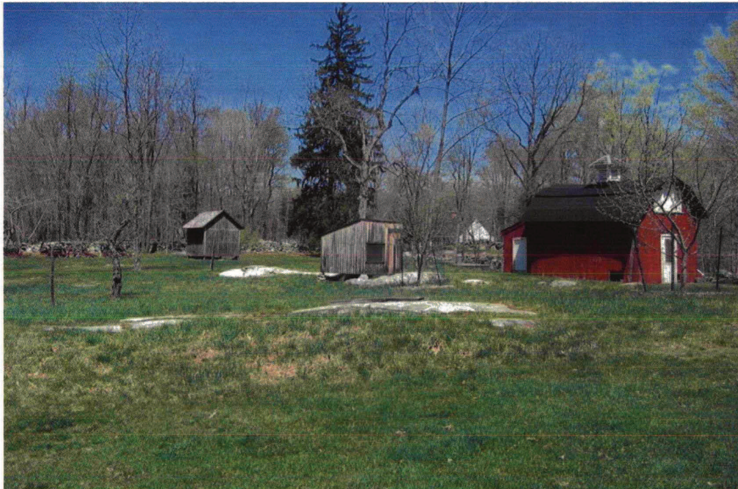
View north (left to right) of the Weir/Young corn crib, animal shelter, and ice house, 2003 (OCLP).
