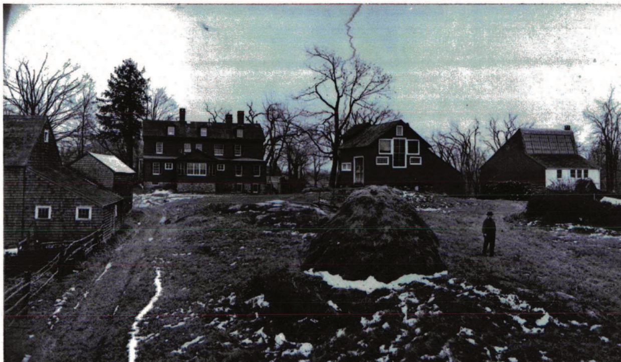
View southwest towards (left to right) Weir/Young barn, Weir/Young house, Weir studio, and Young studio, ca. 1940 (WFNHS-HP No. 150).
