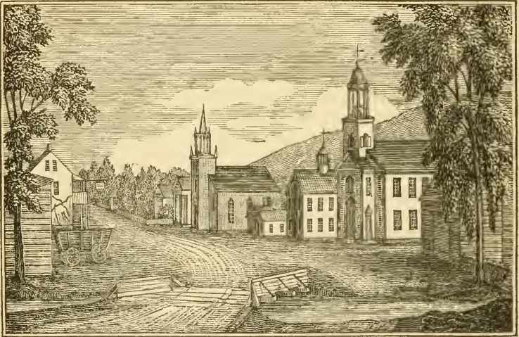
Southwest view of the Churches in Salisbury Center.
