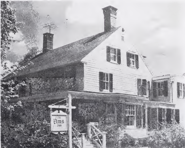
Figure 89 Main Building of the Elms Inn
