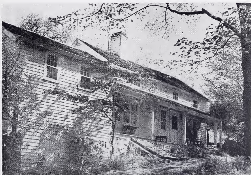
Figure 144 Former Benedict Cobbler Shop
