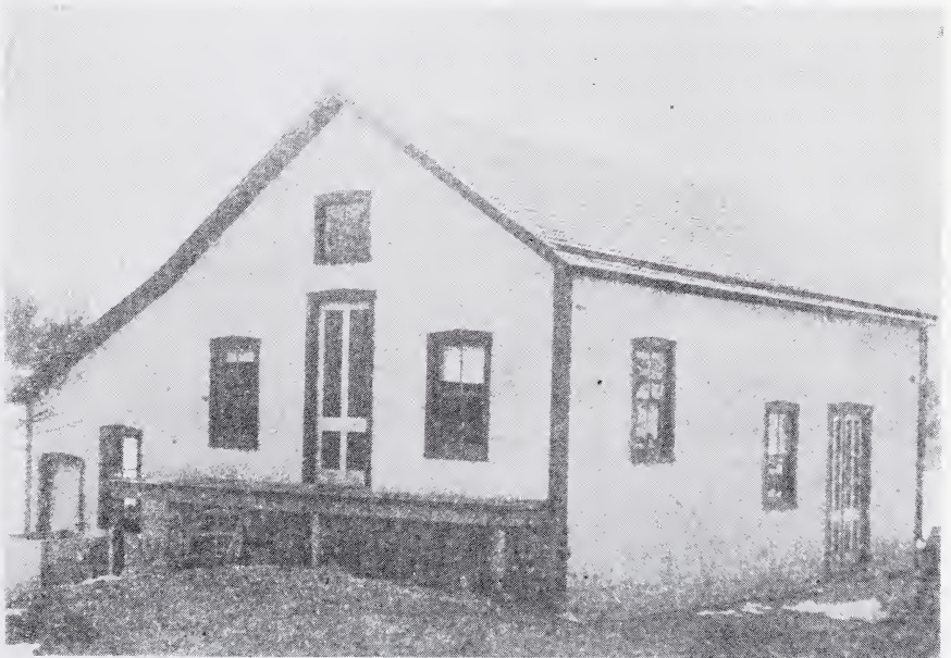
Figure 121 The Creamery Building in about 1900 Believed to have formerly been the Congregational Meeting House
